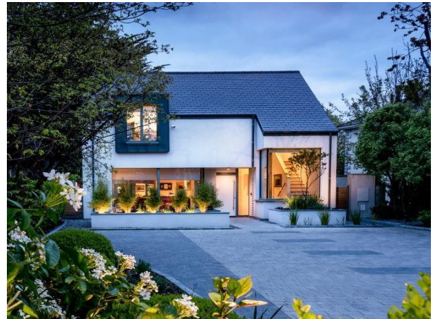
Figure 1: HPI Gold certified passive house at Wayside, Douglas Road, Cork
