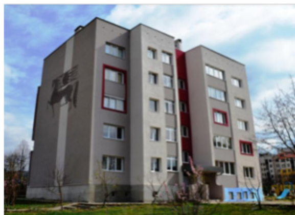
Figure 2: Renovated large panel building in Bulgaria
