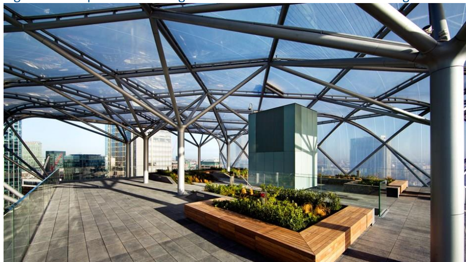
Figure 10: 3D printed cladding 'shrouds' for the Bevis Mark building's roof terrace
