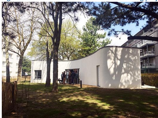
Figure 8: Picture of the YHNOVA social housing project finished in 2018
